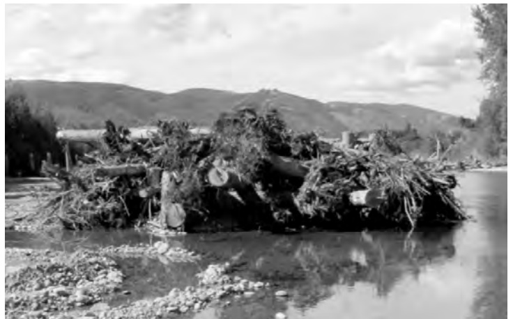
Completed log jam downstream of Hutchinson Creek on the South Fork. ■
