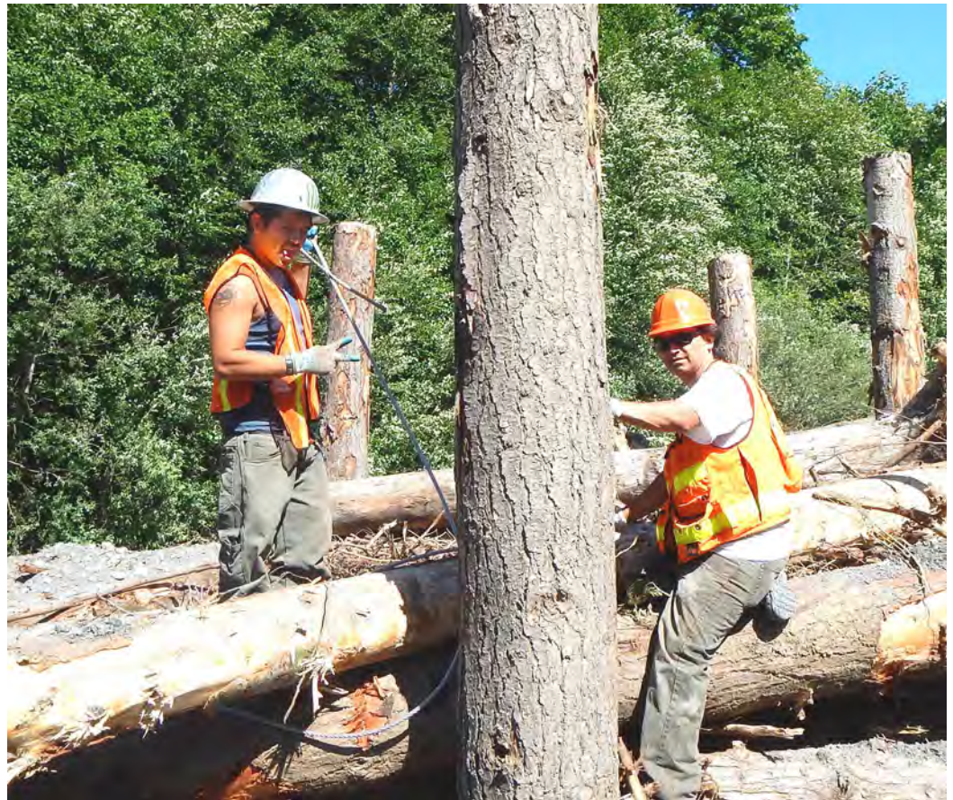
Sindick Bura and Tom Cline tying cable to support log jam.
